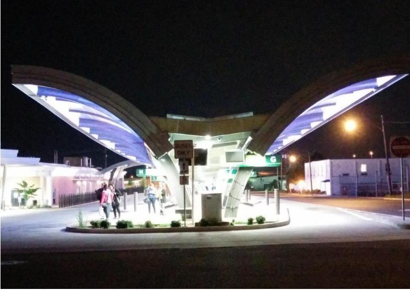
Duo-Gard used its Series 2500 system, engineered for large expanses of sloped glazing. The translucent multiwall polycarbonate in 20mm thickness allows 40% visible light transmittance as it minimizes solar heat gain and glare. The material is shatterproof and completely recyclable.
