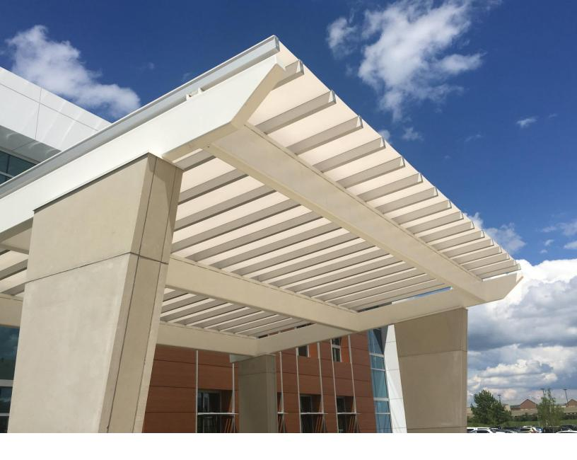
The canopy, from Duo-Gard's award-winning Sleekline Systems, measures 30'6" x 26' and features ¼" panels of white monolithic polycarbonate sheet, framed in clear anodized aluminum. The choice of this translucent glazing material was the design team's solution to the owner's desire for "openness that complemented the glass in the building's renovation," according to Henderson. She adds that the diffused light the canopy provides contributes to a warm, contemporary aesthetic.
