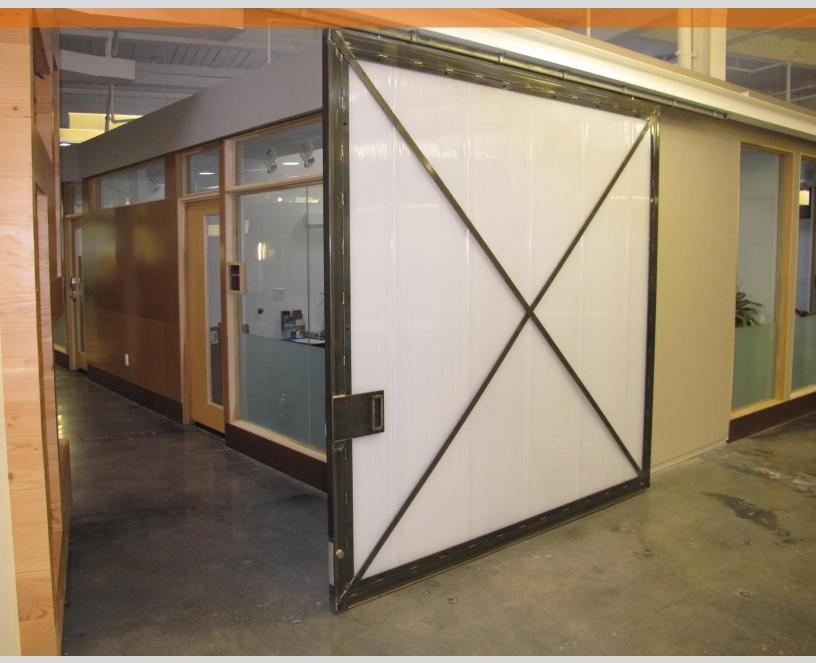
Duo-Gard Industries has created a translucent sliding door system that incorporates 40mm polycarbonate structured sheet available for interior design ideas. The system provides architects and interior designers with a light weight, translucent door applications ranging from warehouse redesign to creating movable office wall solutions.
